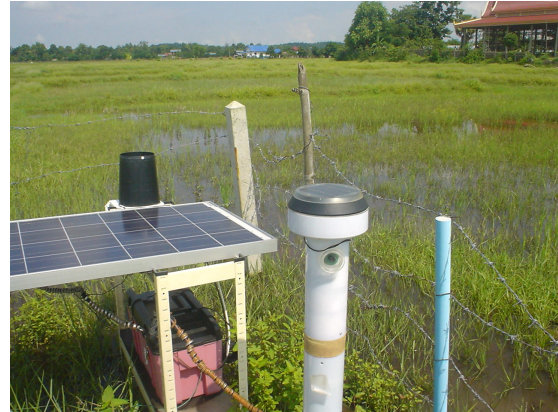
Figure 2. Field Server installed on December 24, 2007.
